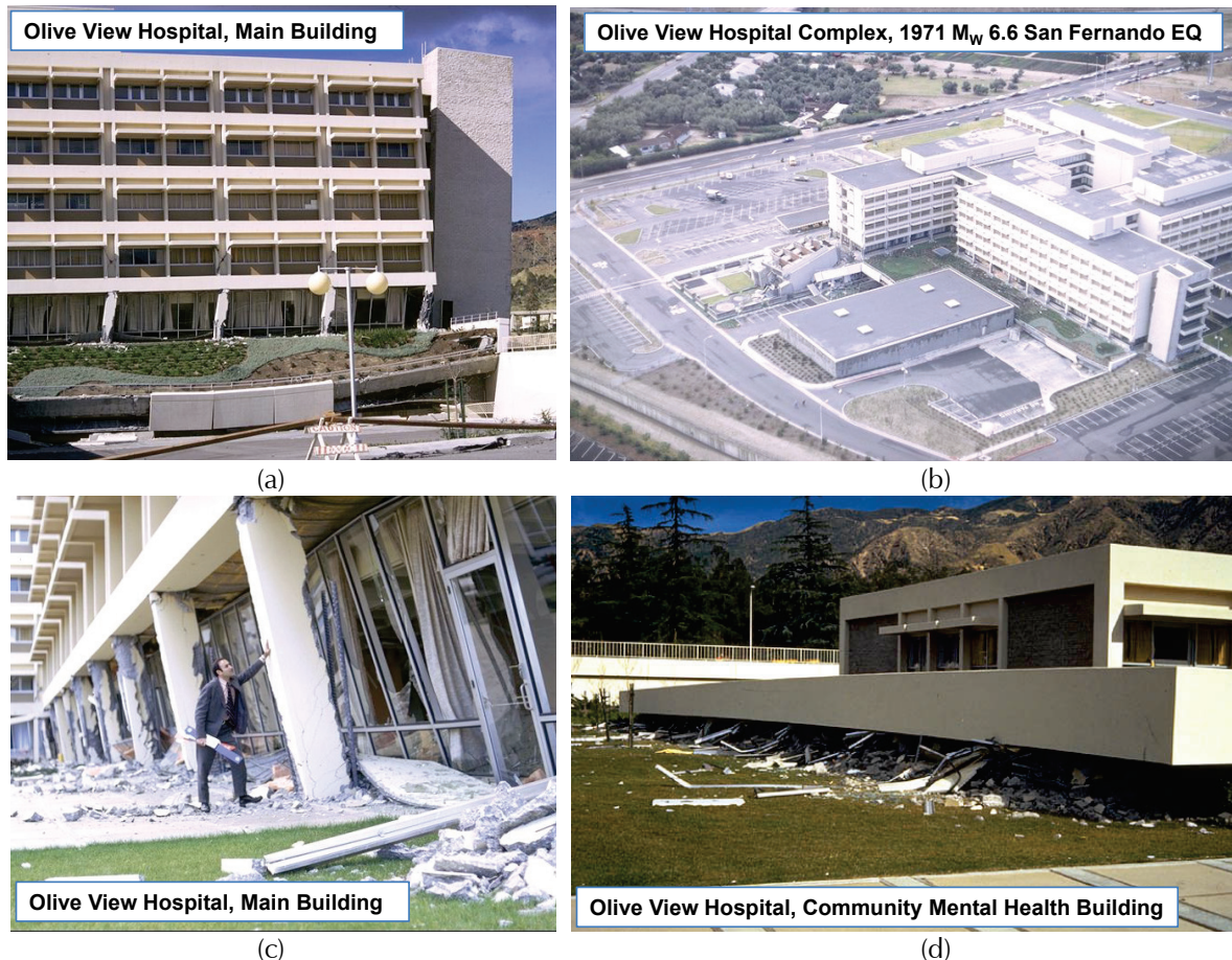
Figure 2-4 Photographs of severe damage and collapse of buildings of the Olive View Hospital due to the 1971 San Fernando earthquake. Photos from NISEE (1971a; 1971b; 1971c; 1971d, respectively).
