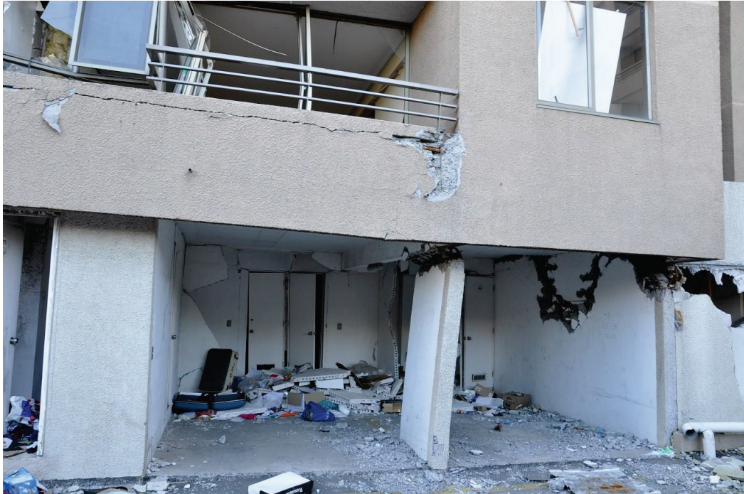
Figure B-2 A change in the wall section from the upper to lower story results in a loss of wall area and localization of flexural yielding (Plaza del Rio Building, Concepción, Chile). Photo courtesy of Ken Elwood.
