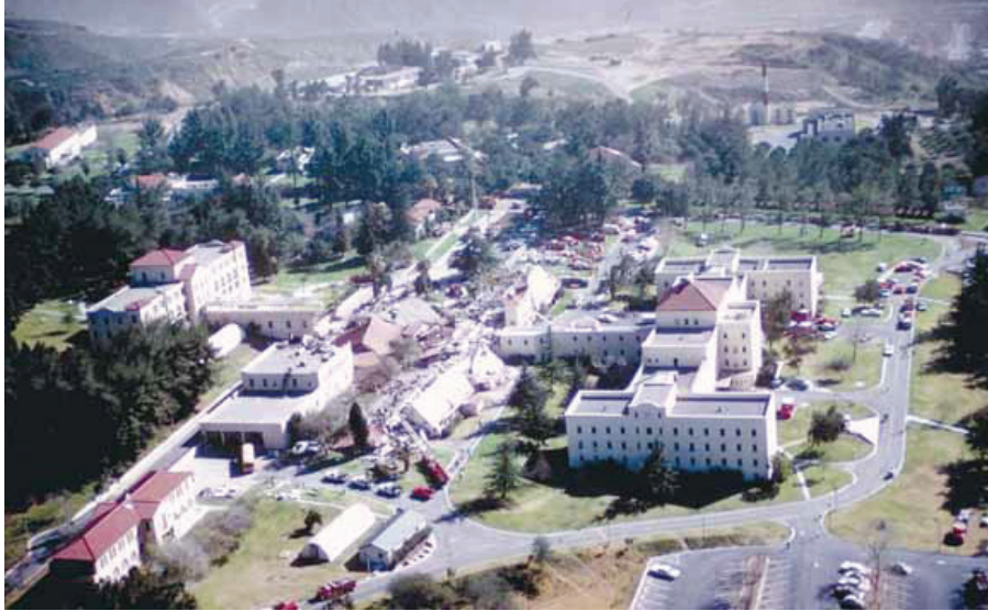
Figure 2-2 Example of non-ductile concrete frame building collapse at the Veterans Administration (VA) complex in the 1971 San Fernando earthquake; including total collapse of 4 of 26 buildings. 47 of the 58 deaths in the 1971 San Fernando earthquake occurred at the VA complex. Photo courtesy of the U.S. Geological Survey.
