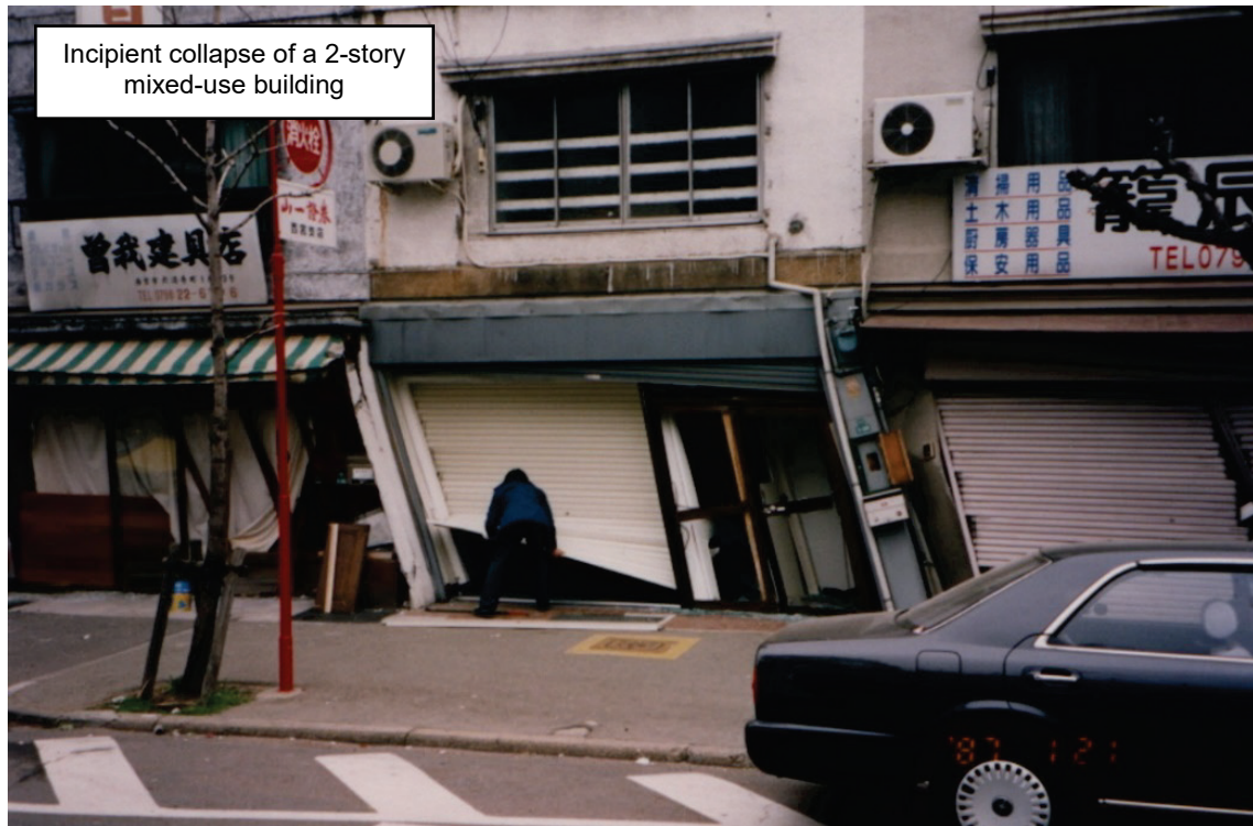
Figure 2-5 Photograph showing severe leaning and incipient collapse of a 2-story mixed-use building in Kobe City. Photo courtesy of Charlie Kircher.
