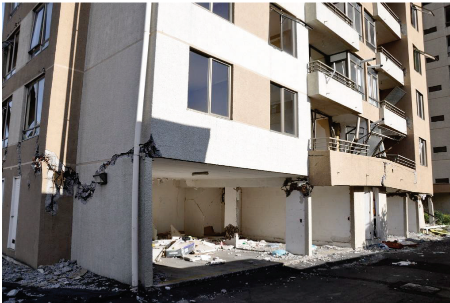
Figure 2-8 Coupled walls in upper stories do not continue to lower story (Plaza del Rio Building, Concepción, Chile). Photo courtesy of Ken Elwood.
