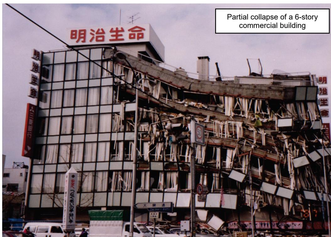
Figure 2-6 Partial collapse of a 6-story commercial building (Chou Ward) with a torsional irregularity. The building was a reinforced concrete structure with perimeter shear walls on two orthogonal sides of the building and gravity framing on the other two orthogonal sides of the building. The torsional irregularity caused the building to rotate during the earthquake. As the building rotated, large displacement of the gravity frames at the corner away from the stiffer walls exceeded frame capacity causing failure of columns and collapse or sagging of floors above. Photo courtesy of Charlie Kircher.
