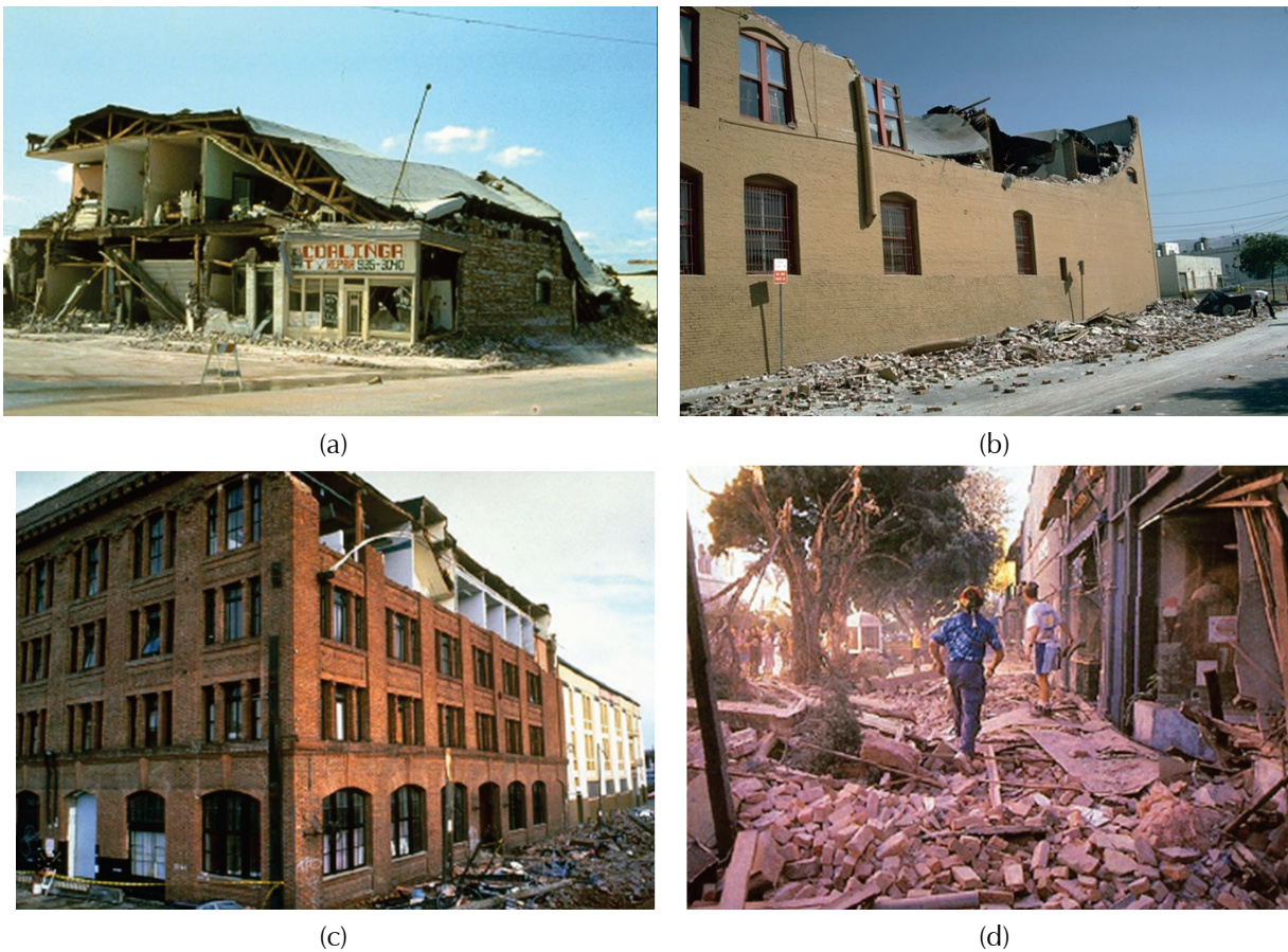
Figure 2-1 Examples of URM building collapse in the (a) 1983 Coalinga earthquake (NISEE, 1983); (b) the 1987 Whittier earthquake (NISEE, 1987), and (c, d) the 1989 Loma Prieta earthquake (photos courtesy of the U.S. Geological Survey and Bill Lovejoy of the Santa Cruz Sentinel, respectively). 5 deaths (San Francisco, photo c) and 3 deaths (Santa Cruz, photo d) out of 15 building collapse-related deaths occurred due to out-of-plane failure of URM walls in the 1989 Loma Prieta earthquake.
