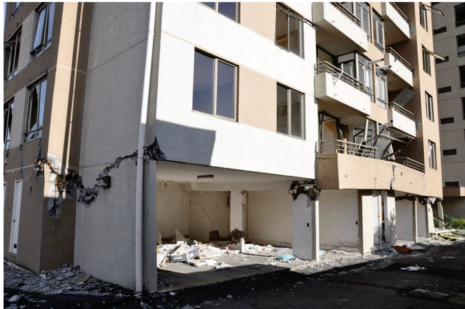
Figure B-1 Coupled walls in upper stories do not continue to lower story (Plaza del Rio Building, Concepción, Chile). Photo courtesy of Ken Elwood.
